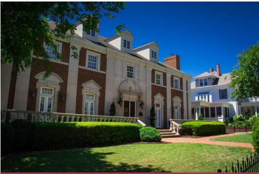
Twickenham Historic District
